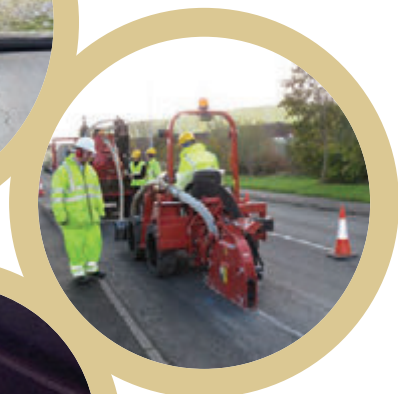
Slot Cutting / Microtrenching
